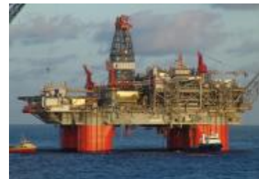
July 18th, professional efforts by a multitude of contractors have rebalanced the platform
